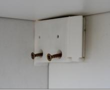
Attatch the cabinet hanging brackets with the 30mm screws provided at the top of the cabinet, where there are pre-positioned holes provided on the side panels for your guidence.
