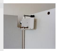
Attatch the cabinet hanging brackets with the 30mm screws provided at the top of the cabinet, where there are pre-positioned holes provided on the side panels for your guidence.
