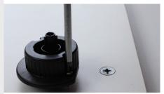
Using a screwdriver secure the socket in position by fixing in two roundhead screws into the holes provided on the socket.
