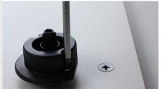
Using a screwdriver secure the socket in position by fixing in two roundhead screws into the holes provided on the socket.
