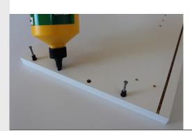
Insert three metal dowels into the holes provided at either end of the side panel and one in the centre as per top image. Prior to inserting apply a small amount of wood PVA glue in the holes.
