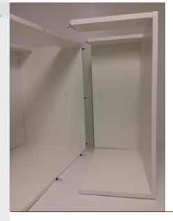
The larger and small cabinets can now be fixed together. Insert the metal dowels into the holes on the larger cabinet, as shown and insert into the corresponding holes on the smaller of the two cabinets.
