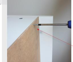
Now insert the back board into the grooves of the side panels. Fix into position using the roundhead screws provided, fixing 5 screws evenly spaced along the top and along the bottom of the back board into the top rail and the bottom panel.
