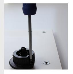
Using a screwdriver secure the socket in position by fixing in two roundhead screws into the holes provided on the socket.
