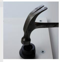
The leg sockets are inserted in to the remaining holes on the underside of the base panel. Twist in and ensure that the flat side of the socket is aligned to the front of the cabinet, leaving the curved edge facing the back. Use a hammer to gently tap in.
