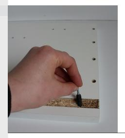
Again using the metal dowels insert one into each of the pre cut holes within the groove on one of the side panels.
