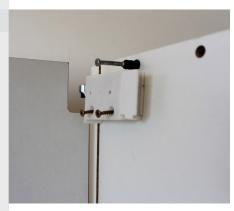
Attatch the cabinet hanging brackets with the 30mm screws provided at the top of the cabinet, where there are pre-positioned holes provided on the side panels for your guidence.
