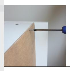
Insert the back panel into the grooves of the side panel. Fix into position using the roundhead screws provided, fixing 3 screws evenly spaced along the top and along the bottom of the panel into the top rail and the bottom panel.
